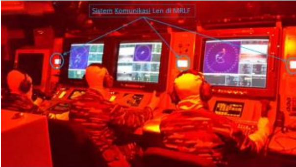
Gambar 11. Naval Intercom System
